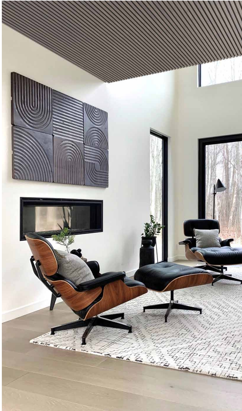
Lamellow Linear Walnut, ceiling installation .
