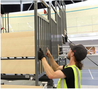
Removable Side Rails - Removed before platforms are retracted and usually stored on a trolley.*
