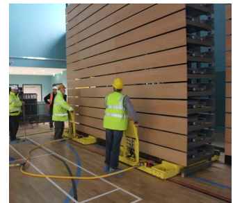
Type M - Mobile. Once closed, units can be specified to be moved via (pictured left to right): a pair of hydraulic trucks, hydraulic trucks with an additional power truck to assist, fork lift truck, or air hover system.
