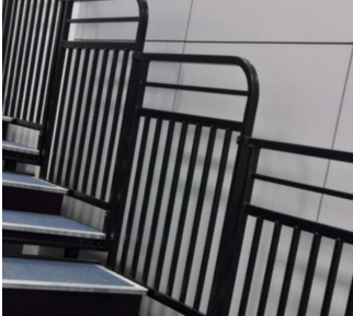
Type D - Tubular steel infill.
