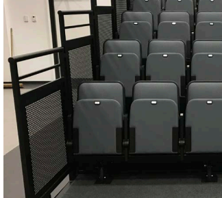
Type E - Perforated steel infill.
