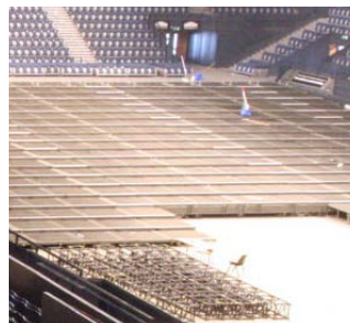
Low Row Rise System - An alternative option where height is restricted. Chairs have to be completely removed before retraction.
