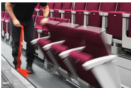
Manual - chairs are folded down in groups of 2, 3 or 4 prior to retraction.
