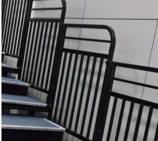
Type D - Tubular steel infill.
