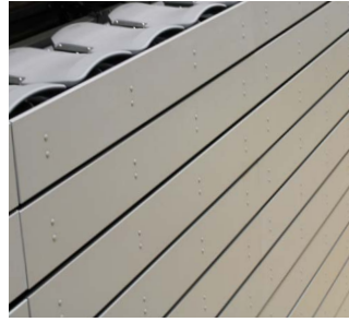
Fascias with plain melamine finish. (Those shown are through bolted for additional strength in a ball sport venue.)
